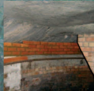
The opening to this pill box at Fairlop Plain in Redbridge was bricked up to prevent people from entering and to minimise drafts. A small gap was left at the top of the brickwork for bats to crawl through. The pill box is situated in a wooded railway sidings that links a country park with fields and allotments.
