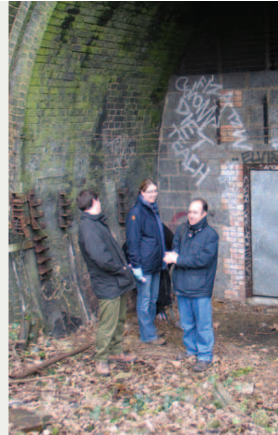
The old railway tunnels close to Highgate Wood in Haringey have been enhanced for bats by building walls to create a more stable internal climate, restricting access for people by the installation of bat friendly grilles and the incorporation of bat hibernation units in the interior.
