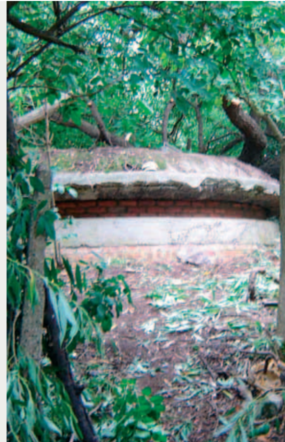
The opening to this pill box at Fairlop Plain in Redbridge was bricked up to prevent people from entering and to minimise drafts. A small gap was left at the top of the brickwork for bats to crawl through. The pill box is situated in a wooded railway sidings that links a country park with fields and allotments.
